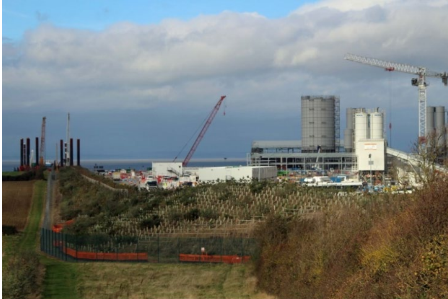
Figure 3. Construction of Hinkley Point Nuclear Power Station
